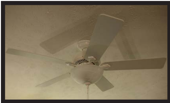
Upgrade Ceiling Fan
