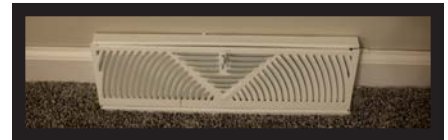
Perimeter Heat Wall Mount Register
