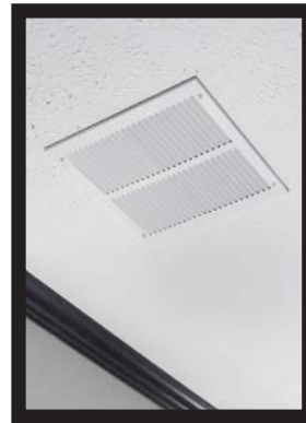
Return Air in Ceilings w/ Lower Interior Doors (HUD 5/12 - Bedrooms Only)
